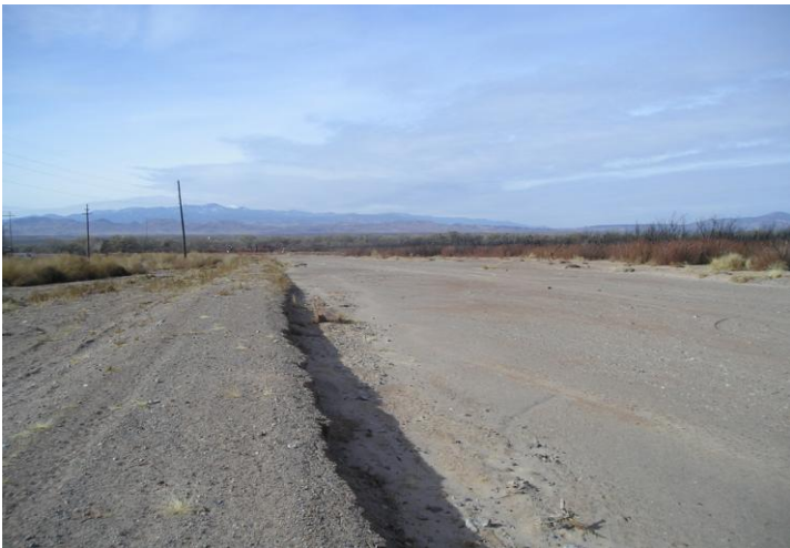
Dike constructed by Socorro County - looking west
